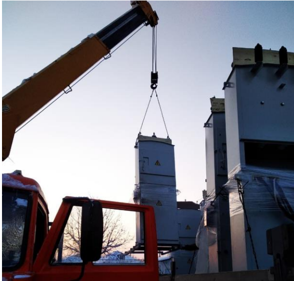
Figure 24. Installing power transformers in the pilot regions.
