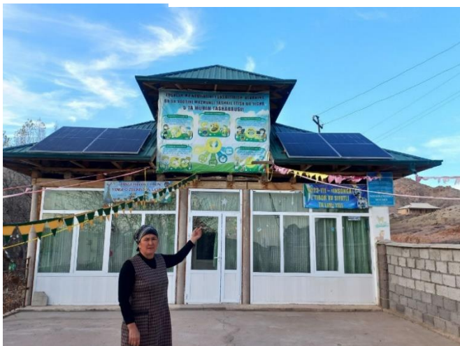
Figure 32. Solar panels for Kindergarten (Charkesar).
