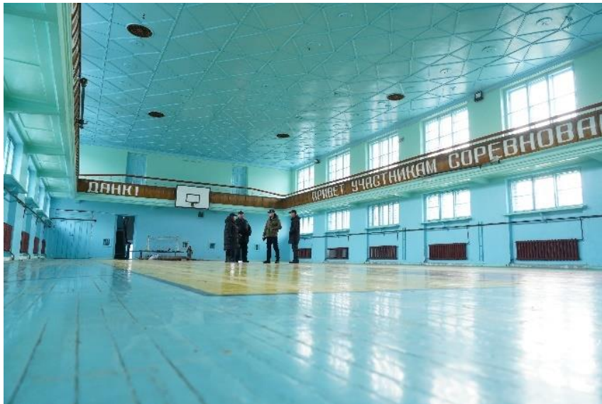
Figure 18. Heating system of the city gym in Mailuu-Suu was repaired.
