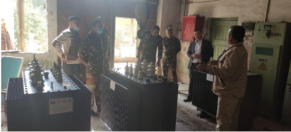
Figure 35. Site visits conducted to visit the power transformers installed.
